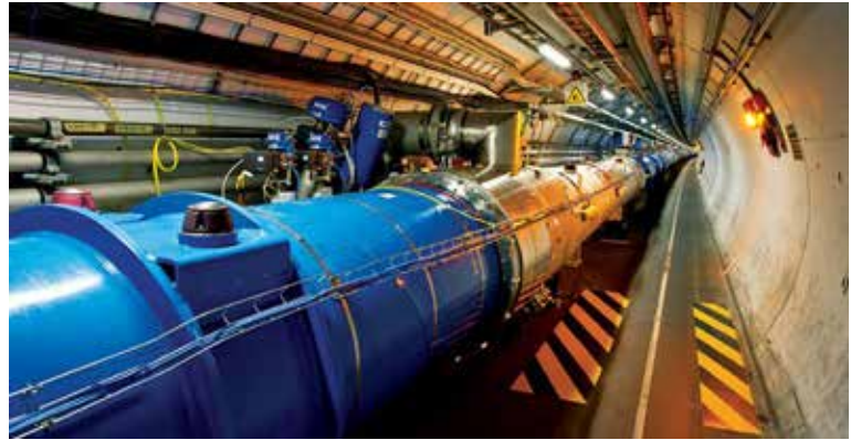
Figure 6 The LHC tunnel, where beams of particles pass through central pipes before colliding with each other. [Credit: CERN]
