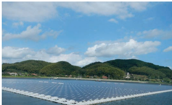
Figure 3 (left) In Japan, solar arrays floating on water take advantage of open water where land space is constrained.
