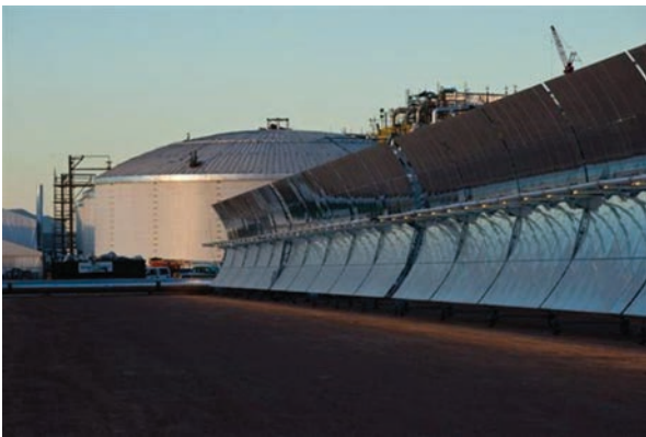
Figure 7 Thermal storage tank and some of the parabolic trough mirrors.
