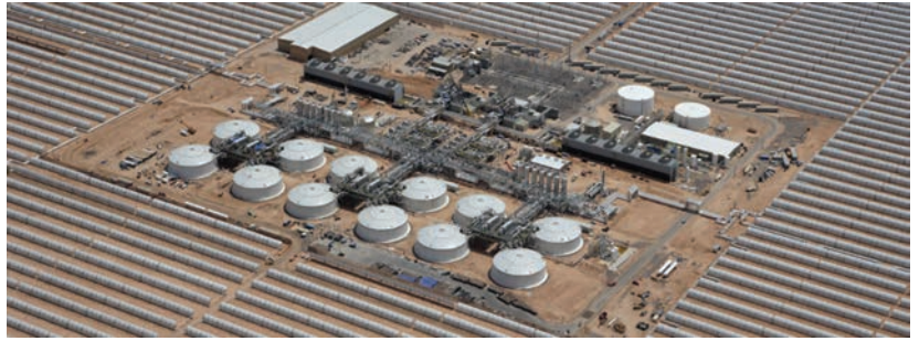
Figure 6 Aerial view of the power block at Solana Solar Generating Station, surrounded by its mirrors.
